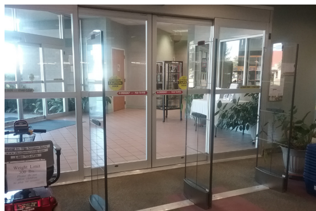
DeRidder branch automatic doors and security gate
